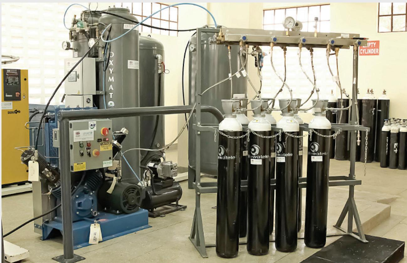
**Exhibit 2:** PSA systems typically have two adsorption beds, which alternate between adsorbing nitrogen from air while allowing oxygen to flow through, and venting the accumulated nitrogen into the atmosphere. VSA uses the same general principle but operates at lower (vacuum) pressures. The photograph shows a typical PSA facility filling cylinders. (Courtesy: Hewatele, Kenya)
