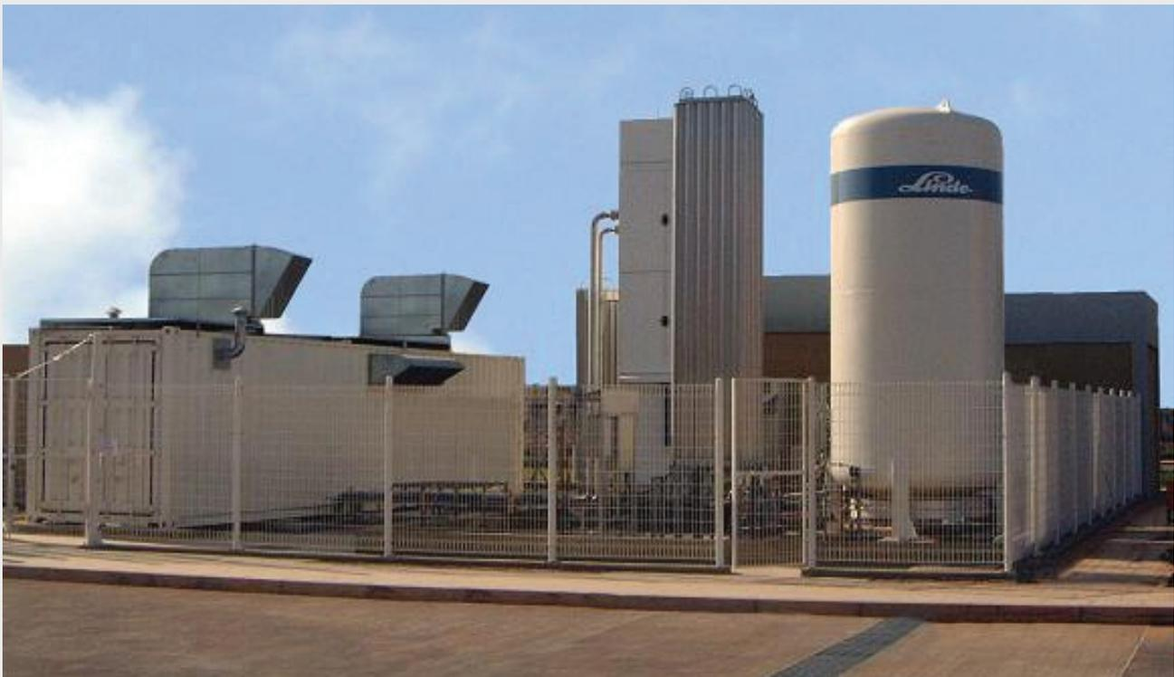
**Exhibit 1:** Cryogenic air separation begins by compressing and purifying ambient air, followed by liquification and fractional distillation to separate oxygen from other components. The resulting liquid oxygen (LOX) is >99.5% pure, well above what is needed for medical treatment. The photograph shows a typical LOX plant.
